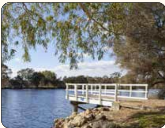
Deck Structure (River Access)
