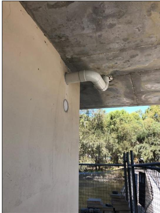
*Figure 4: Minor drainage pipe encroachment*
