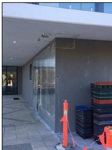
*Figure 4: Removal of minor drainage pipe encroachment*
