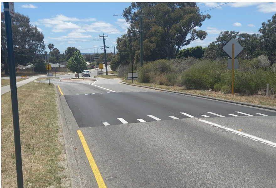
Stanton Road: Raised plateau traffic calming treatment view towards Kanowna Avenue on the left.
