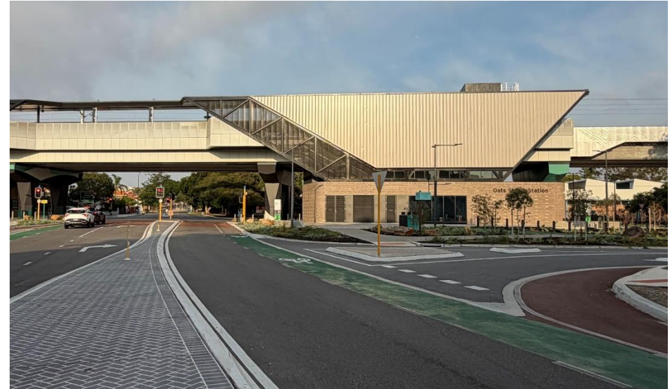
Oats Street Station, a potential destination for City residents to ride to. Source: City of Belmont
