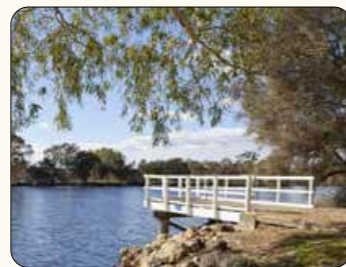
4 Deck Structure (River Access)
