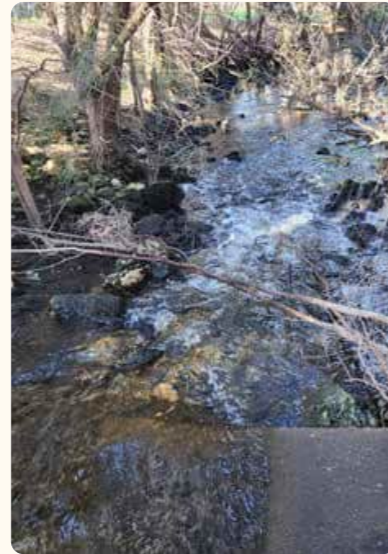
Drain / Channel Character
