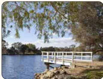
Deck Structure (River Access)
