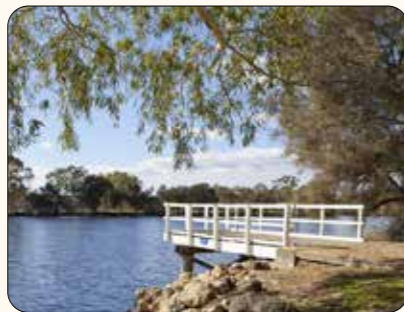
4 Deck Structure (River Access)
