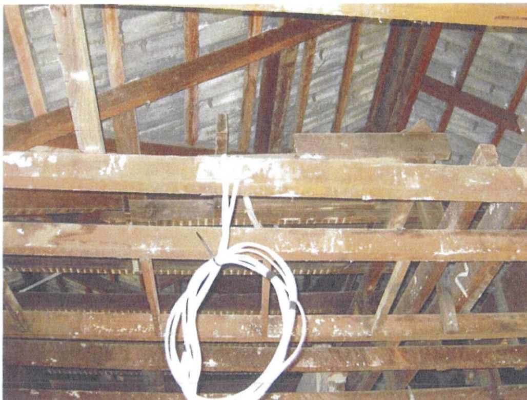
Roof timbers and additional bracing.
