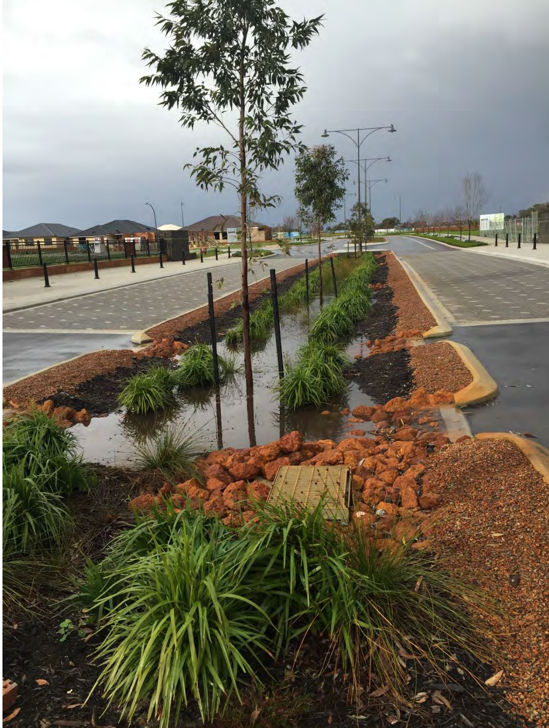
Figure 13: Typical median swale or biofilter
