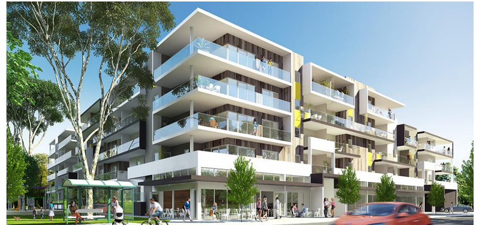
Above: Example of 5 storey mixed use building featuring retail/food and beverage uses at the ground level and residential living above producing a sustainable and active development outcome. In addition, this illustrates the beneficial outcome for buildings to interact with key mature trees available within the proposed Golden Gateway public realm.
