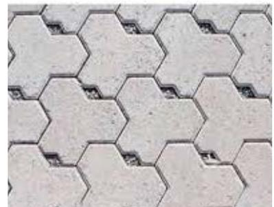
Example: Permeable concrete interlocking pavements
