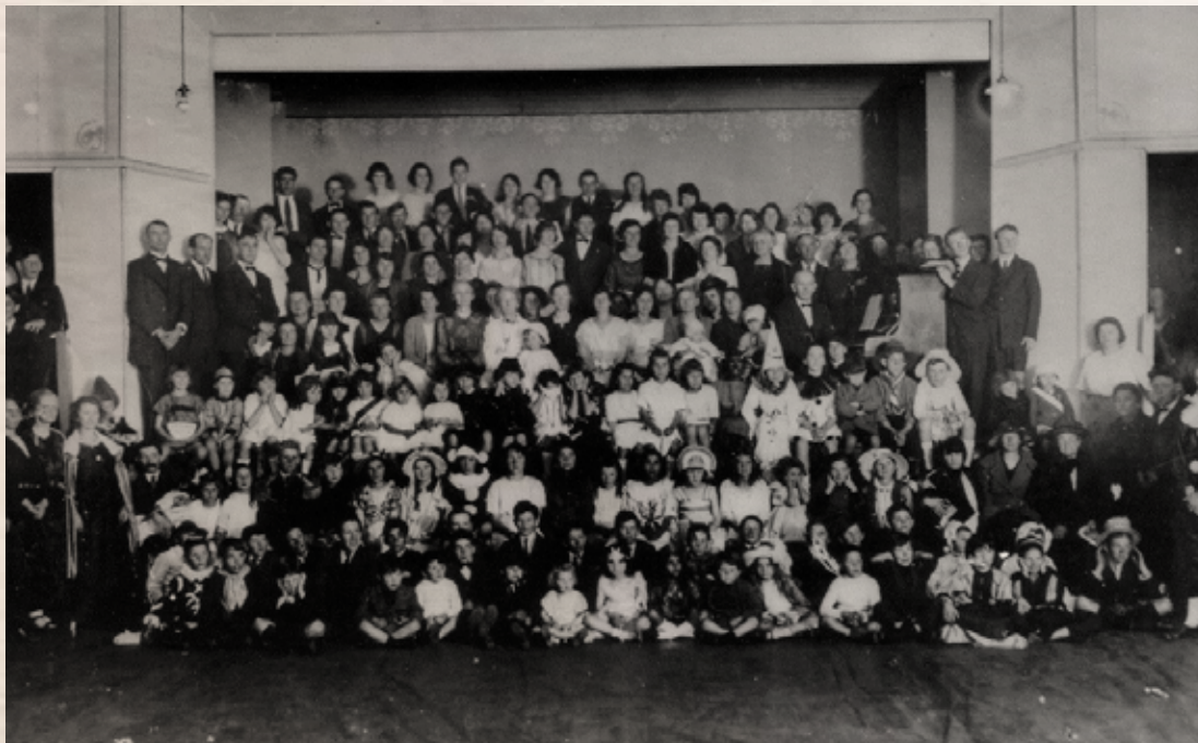
Riversdale Hall interior
