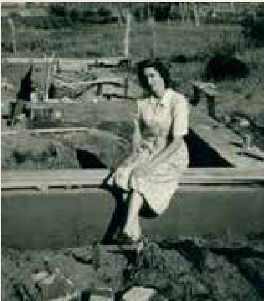
Doreen Ahrens seated on front bedroom foundations: 1950
