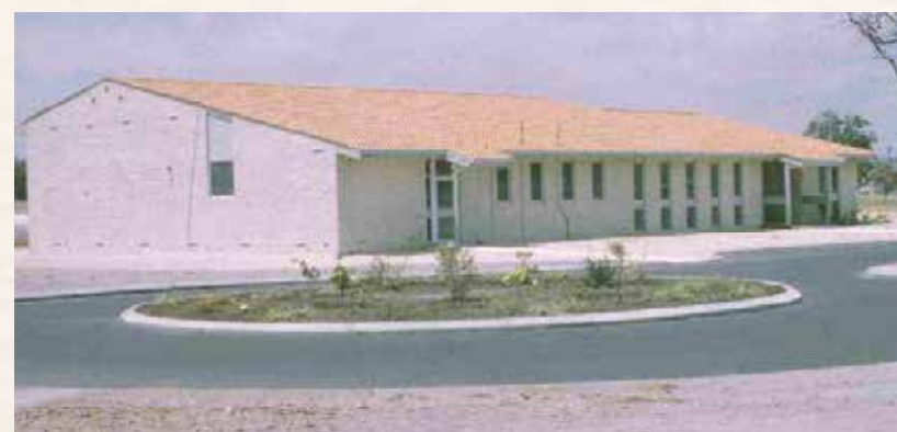
Belmont Senior Citizens Centre under construction, Faulkner Park (1971)
