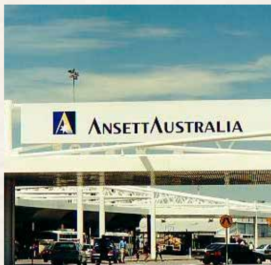
Perth Domestic Airport (2000)
