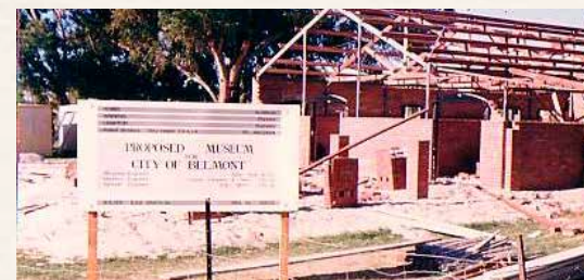
Belmont Museum under construction (1988)
