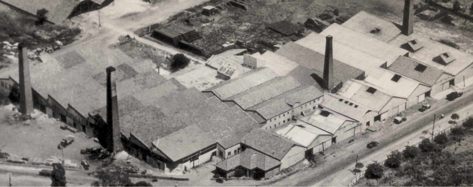
Aerial view of Bristle Factory (1940s)
