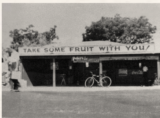
Barrington's Store, 55 Great Eastern Highway, near Belmont Avenue (1930s)
