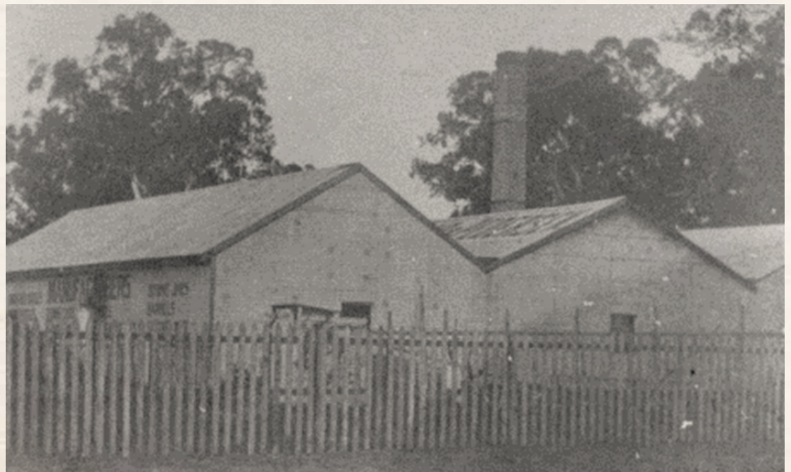
Original buildings – Courtland Pottery
