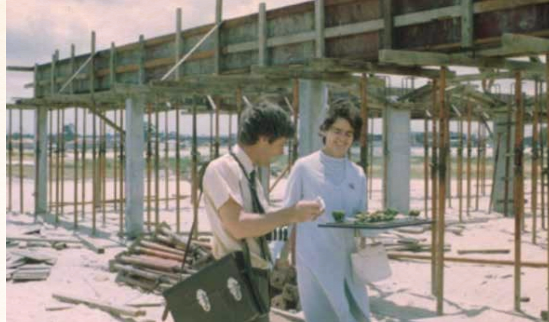
Councillor Ruth Faulkner at the construction site of the public library (1970)
