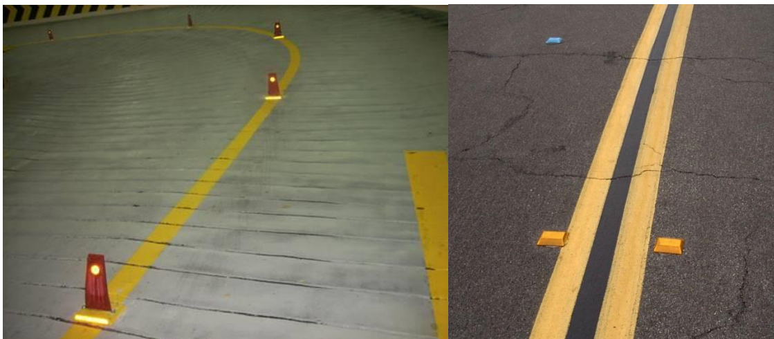
Figure 6: Examples of Pavement Flap and RRPM Devices
