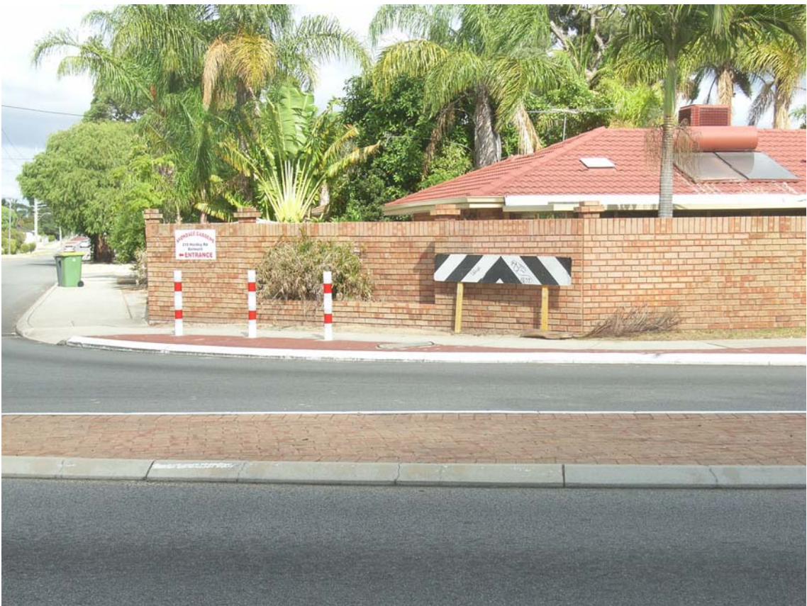
PHOTO 8 North-west corner. Hazard board not facing any oncoming traffic.
