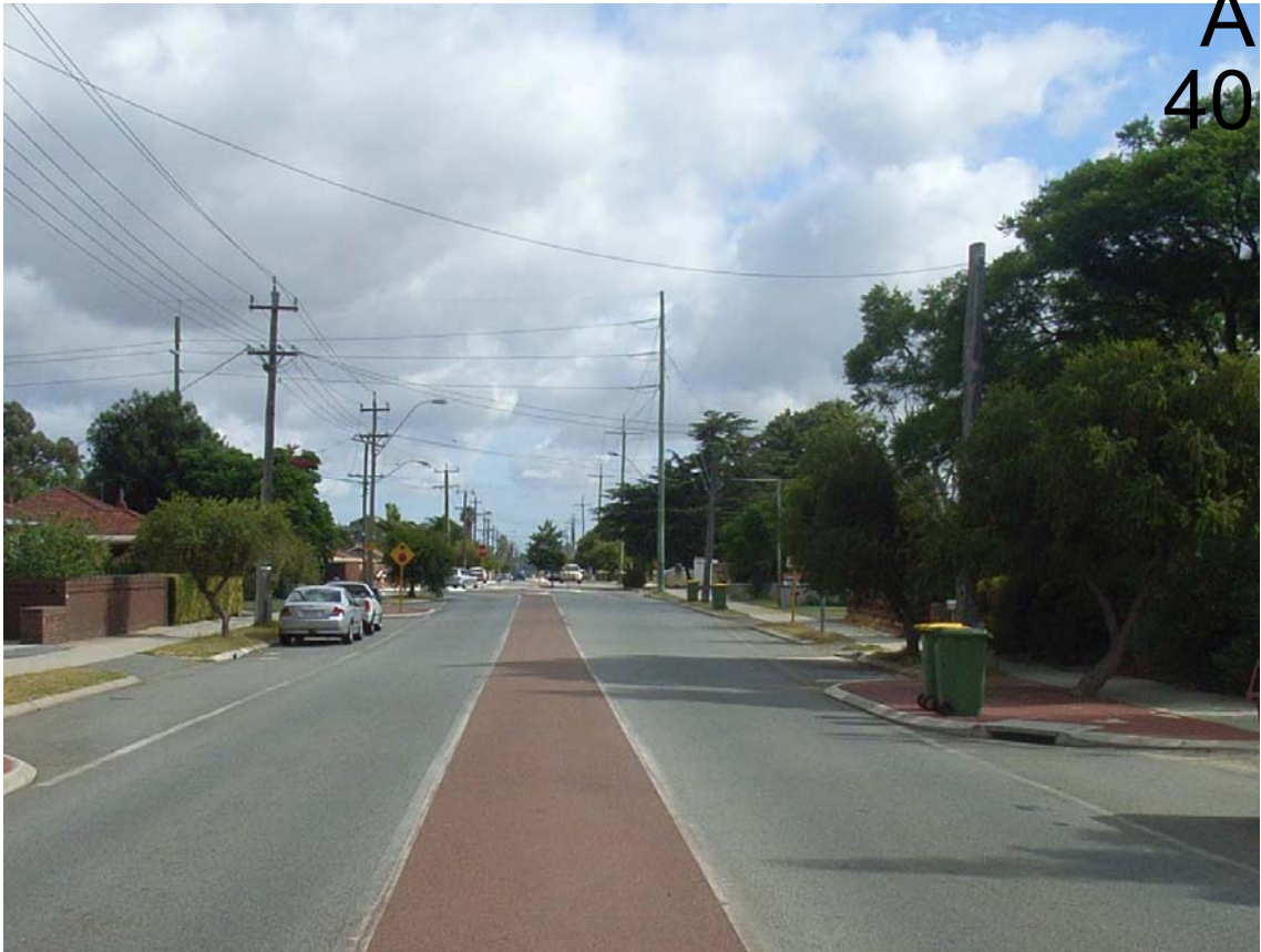
PHOTO 7 Hardey Rd south approach. Wide road with no vertical elements not conducive to lower speeds.
