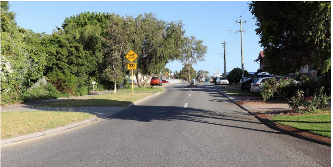
Figure 8: Fauntleroy Avenue looking south from Hay Road
