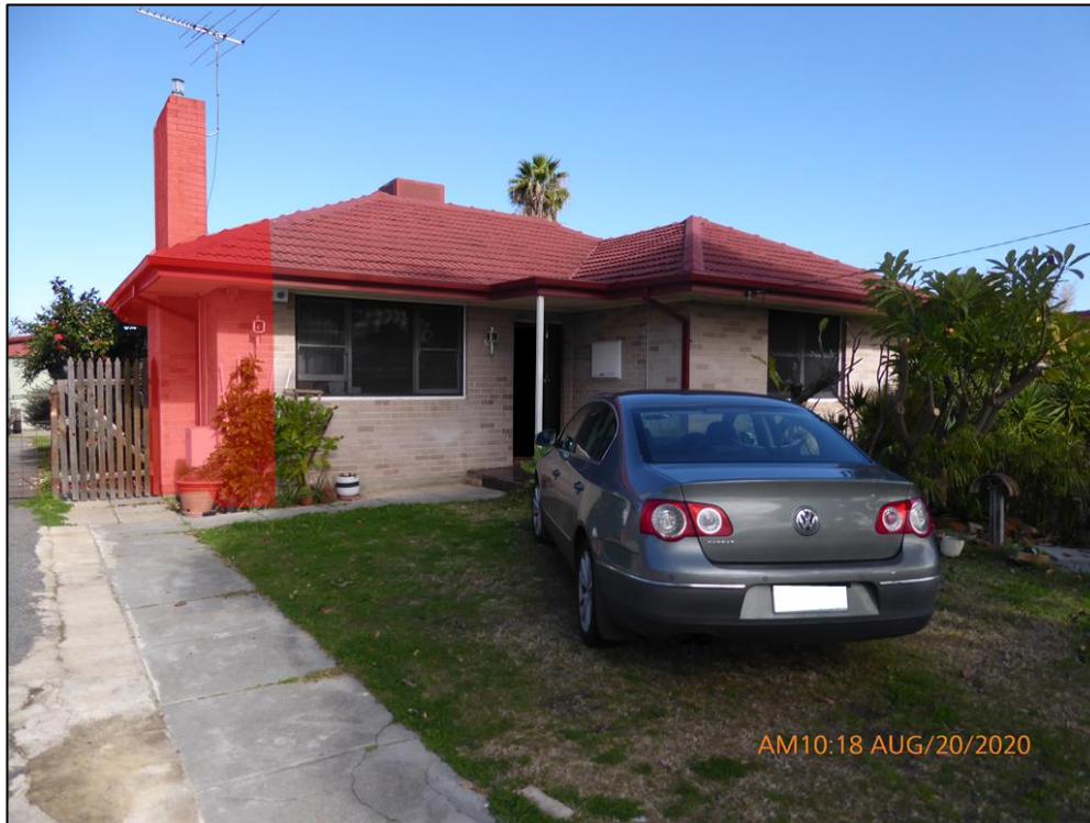
Figure 8: Portion of Existing House Requiring Demolition to Comply with Clause 5.7.3(c) of LPS 15
