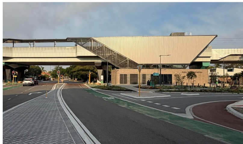
Oats Street Station, a potential destination for City residents to ride to. Source: City of Belmont
