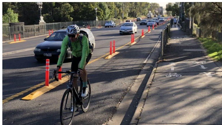
Pop-up bicycle lane in Melbourne. Source: Bicycle Network
