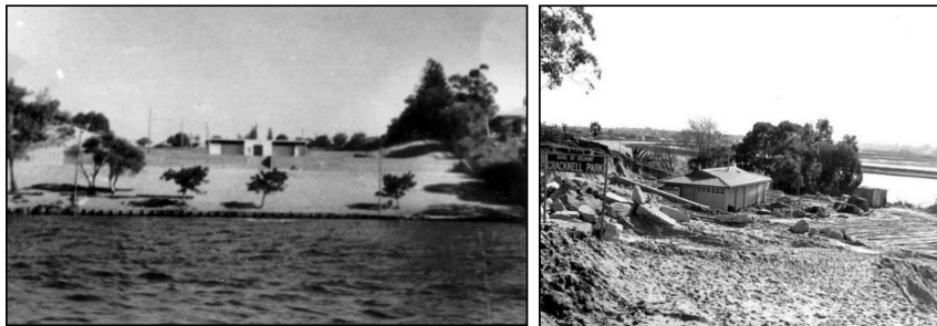
Figure 24: Left: Cracknell Park, Rivervale, circa 1950. Right: Cracknell under construction circa 2000 (right).
