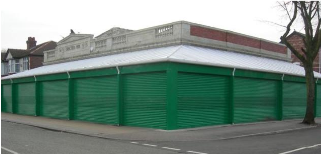
Figure 3: Example of Solid Roller Shutters that will not be supported by the City.
