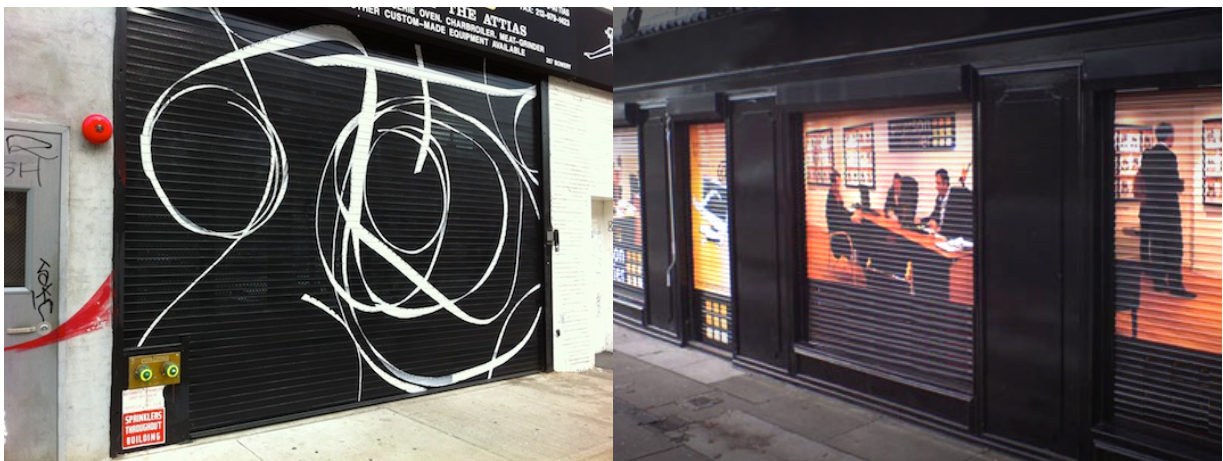
Figure 2: Examples of Roller Shutters that incorporate a decorative graphic design which relates directly to the business.
